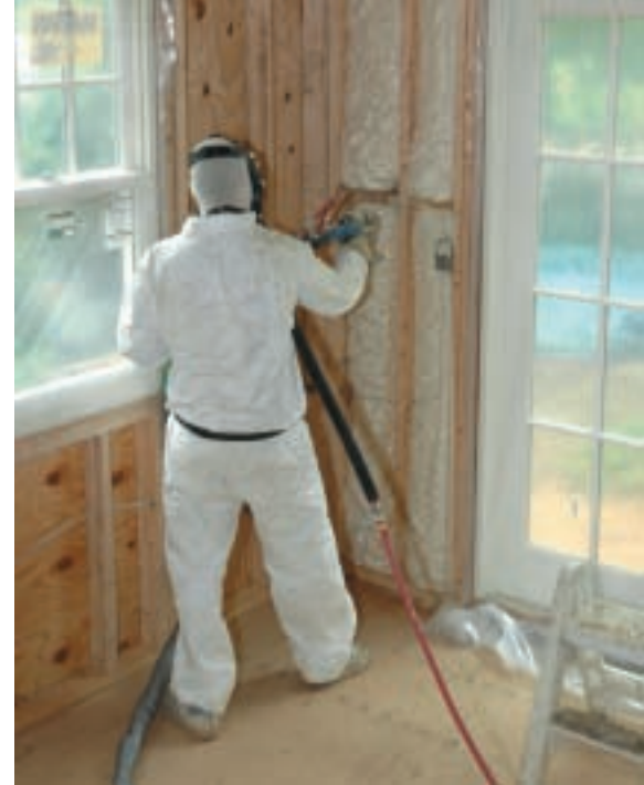
Two Fayetteville fire stations are now insulated with a soy-based spray foam insulation. Success with the product is leading to its use in local court buildings as well as commercial buildings and more.
