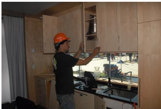
Virginia Tech team member Corey McCalla inspects cabinets made with plywood that uses soy as a bonding agent that does not emit harmful fumes from urea formaldehyde.
