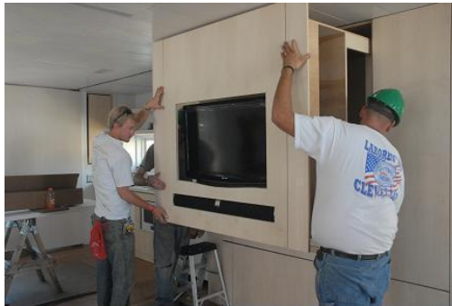
The Ohio State team members install a wall unit.
